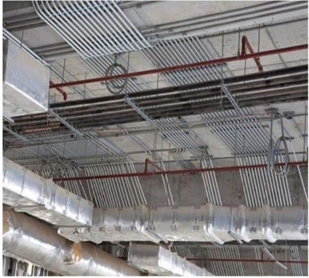
EMT ELECTRICAL SYSTEMS LAY OUT
