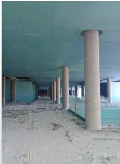
Installation Gypsum board
