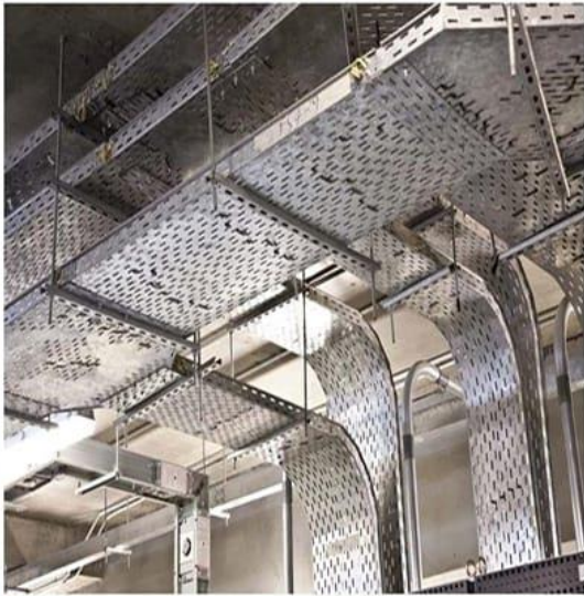
CABLE TRAYS ELECTRICAL SYSTEMS WORKS
