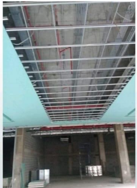
Installation Gypsum board
