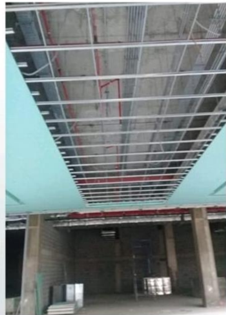
Installation Gypsum board
